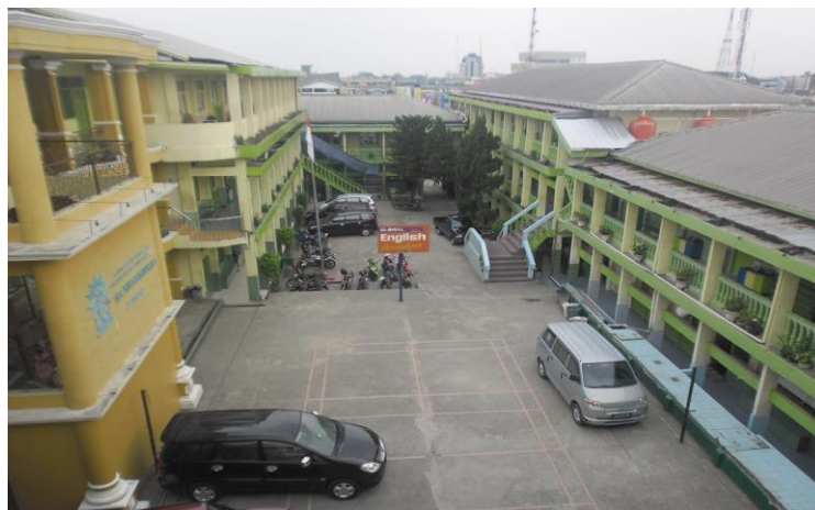
Gambar 8: Gedung A KH. Ahmad Dahlan
