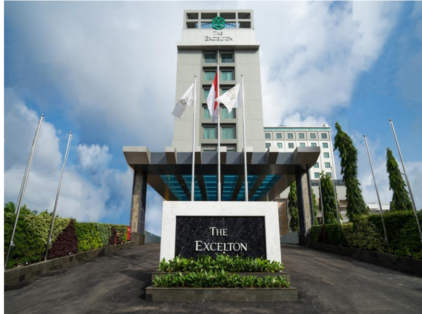
Gambar 1. Gedung Hotel The Excelton Palembang
